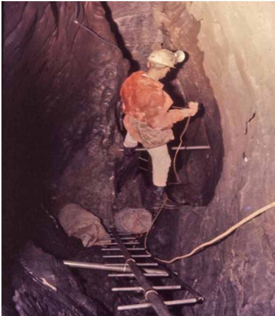
Fixed Ladders Fig13
